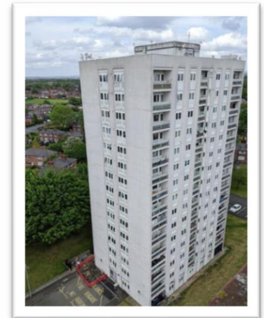
Newton Heath: Avro Hollows Tower Block 2 to be included in SHDF programme.
